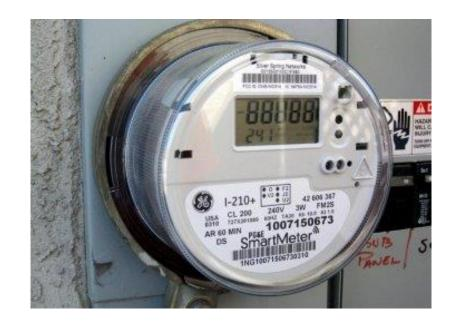
$$\frac{250 \text{ bytes}}{4 \text{ hours}} * 370000 \text{ devices} \approx \frac{51000 \text{ bps}}{120 \text{ km}^2} \approx 1.5 \frac{bph}{m^2}$$
